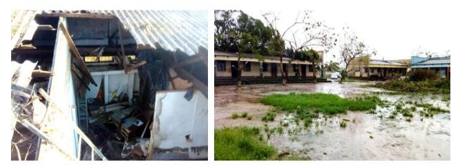
As well as the dormitory, there was damage to the roofs and windows of the classroom blocks and the new kitchen/dining room that was under construction had the roof fully peeled off by the high winds.
